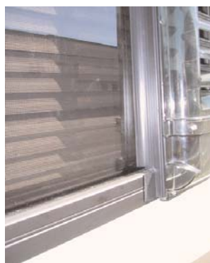
Cut Wiper Gasket FIG T
