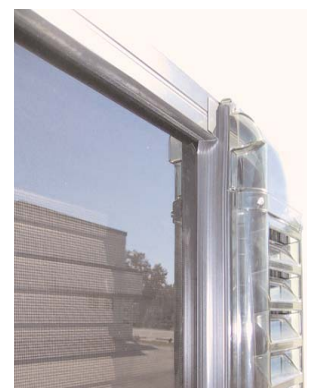
Cut Wiper Gasket FIG T
